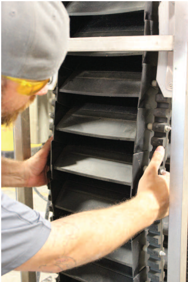
An operator inspects this bucket elevator's drive belts and bucket assembly for signs of wear or damage.
