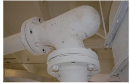
***This flanged 90-degree elbow has functioned in the pebble-lime conveying line without problems for more than 5 years.***
