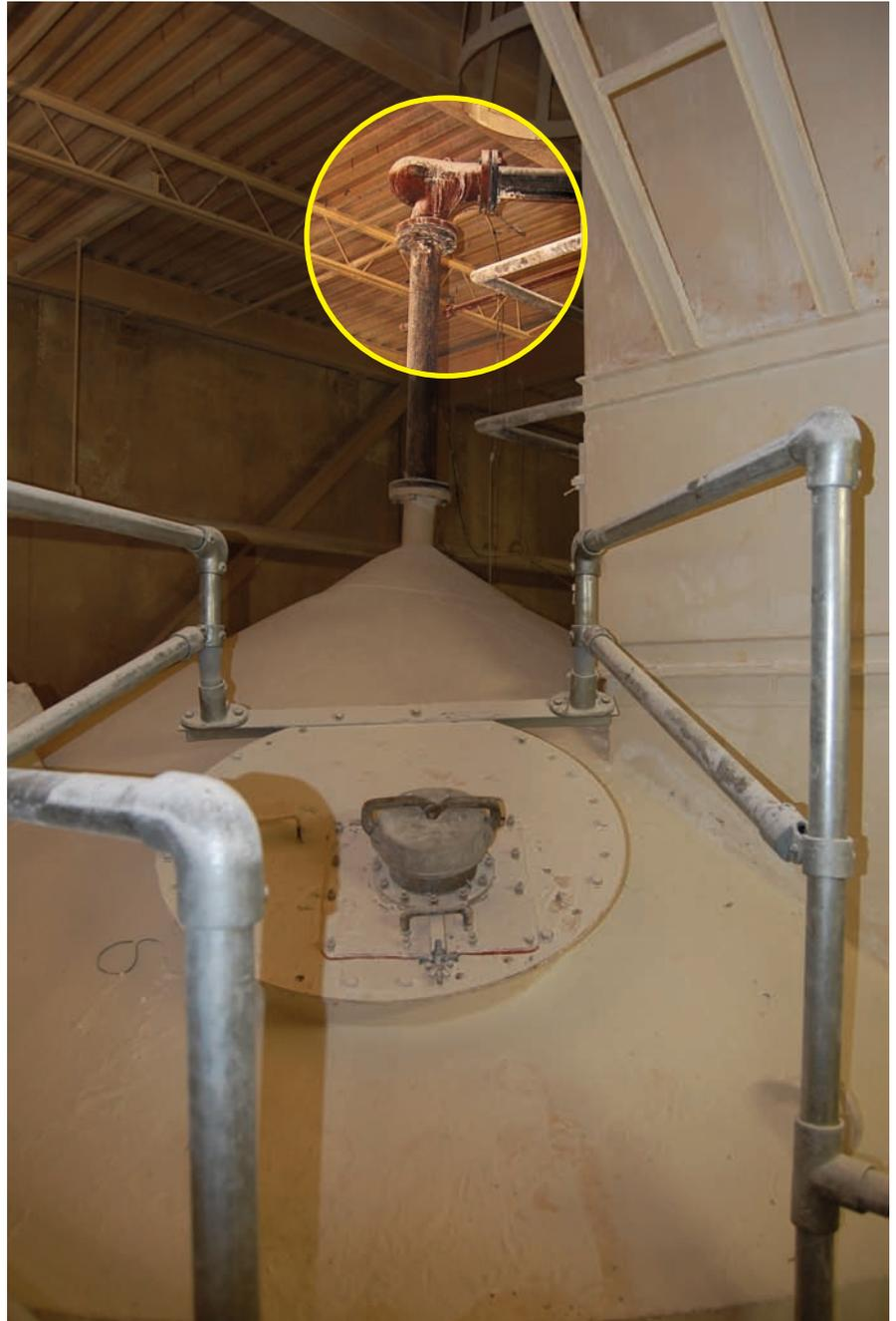
*To reduce maintenance costs and worries, the company installed a new 90-degree elbow (shown in the highlighted area) in a conveying line to direct the pebble lime into a silo's top.*
